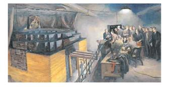
The fuel was lumps of Uranium embedded in blocks of graphite.
